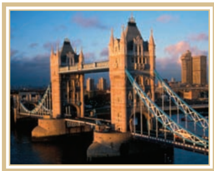
Tower Bridge, London, England
