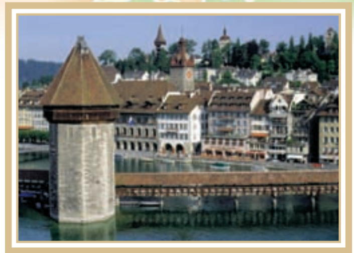
Chapel Bridge, Lucerne, Switzerland
