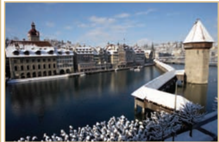
Chapel Bridge, Lucerne, Switzerland
